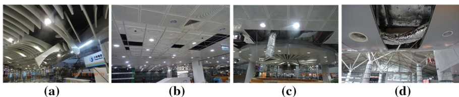
Fig. 19 a Fallen baffle boards, b fallen metal ceilings, c a ventilation duct hanging through the hole where the ceilings fell, and d a damaged sprinkler pipe used for fire-fighting in an airport terminal
