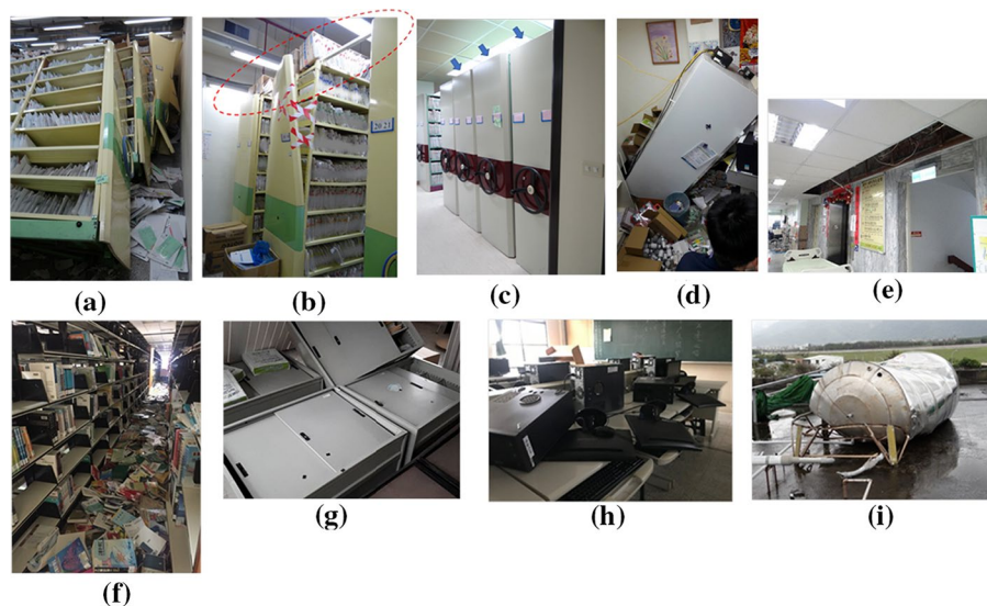
Fig. 18 a–c Damaged shelves for medical history sheets in a hospital. d An overturned medicine refrigerator. e Fallen ceilings in a hospital. f Books fallen from bookshelves. Overturned g filing cabinets and h desk computers. i A damaged water storage tank
