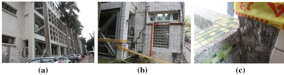
Fig. 16 a and b Cracked brick walls. c A cracked column of a four-story school building
